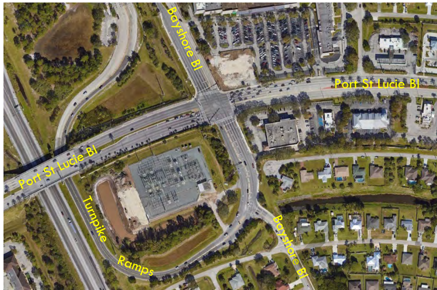
Figure 5.3 Port St Lucie Blvd at Bayshore Blvd
