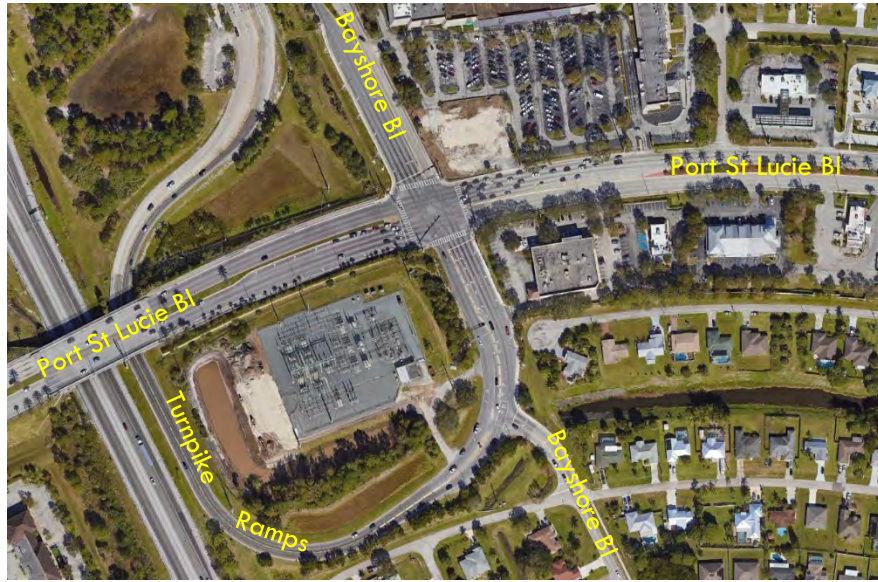
Figure 5.3 Port St Lucie Blvd at Bayshore Blvd
