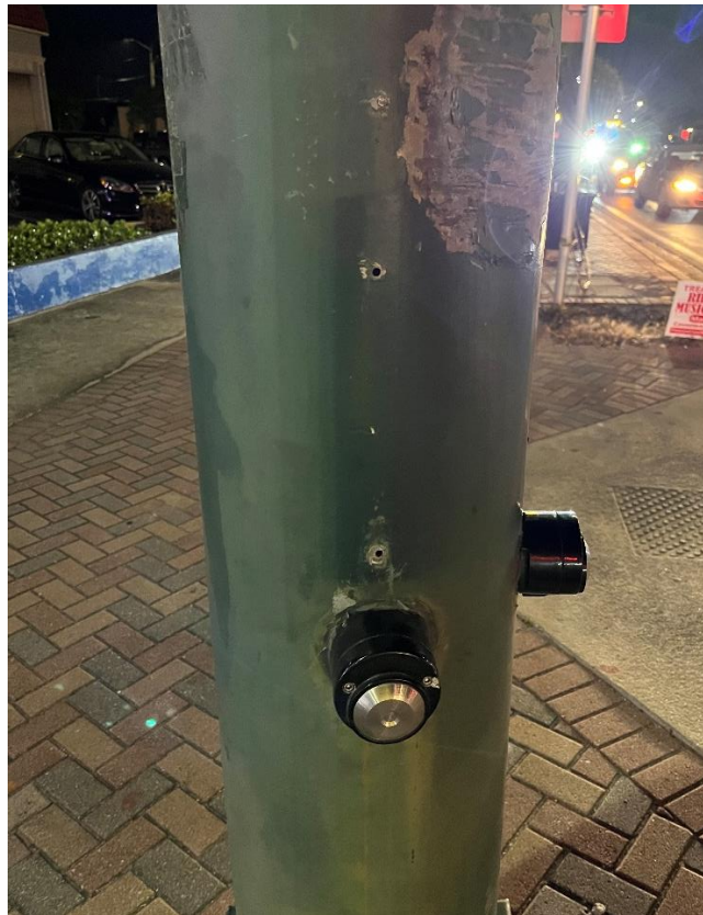
Exhibit 33: Missing Pedestrian Traffic Signal (Walk/Don't Walk) Signs
