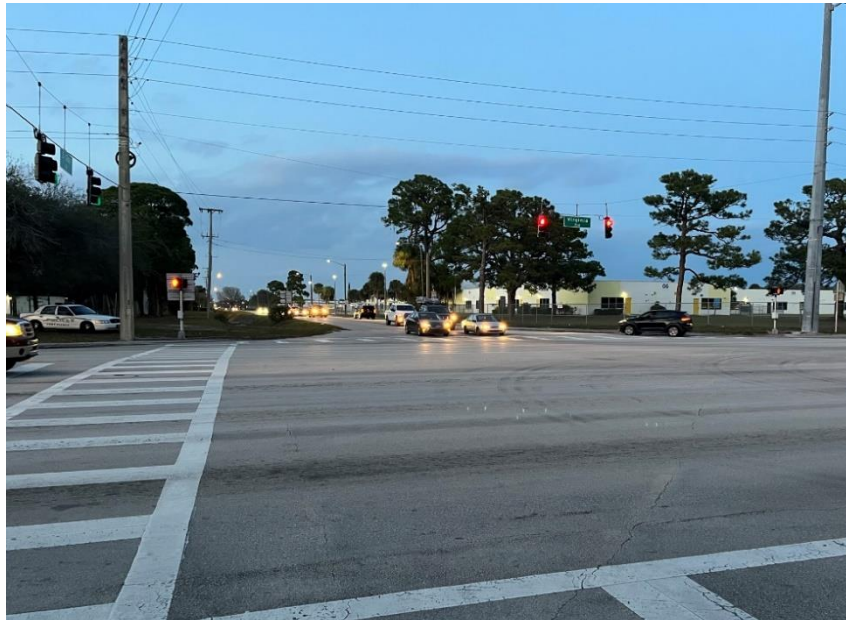
Exhibit 48: S 13 th Street and Virginia Avenue Intersection
