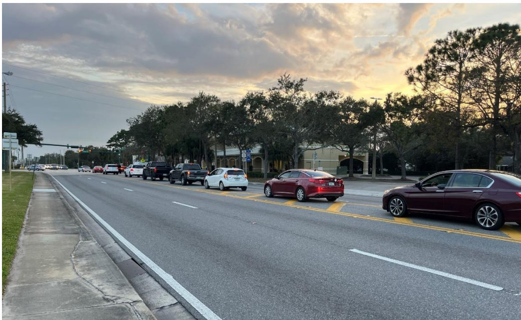
Exhibit 47: Southbound Left Turn Spillback onto Taper
