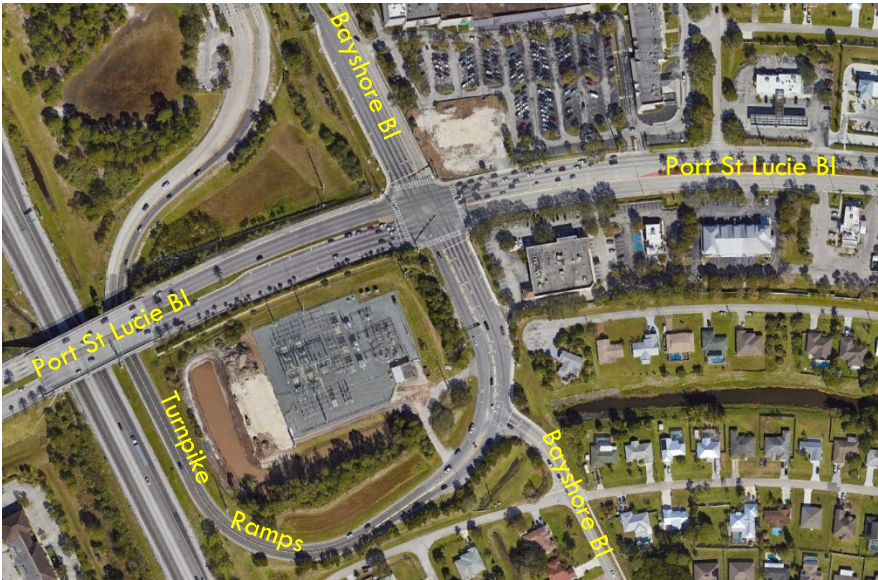
Figure 5.3 Port St Lucie Blvd at Bayshore Blvd
