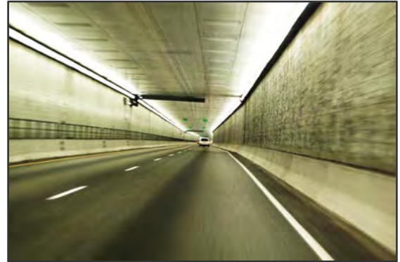
Figure 2-2: View from Inside the Eisenhower Tunnel
